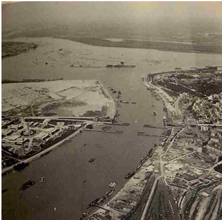
Figure 29: Construction of Gazela bridge on river Sava, 1966, Courtesy of www.wikipedia.org
