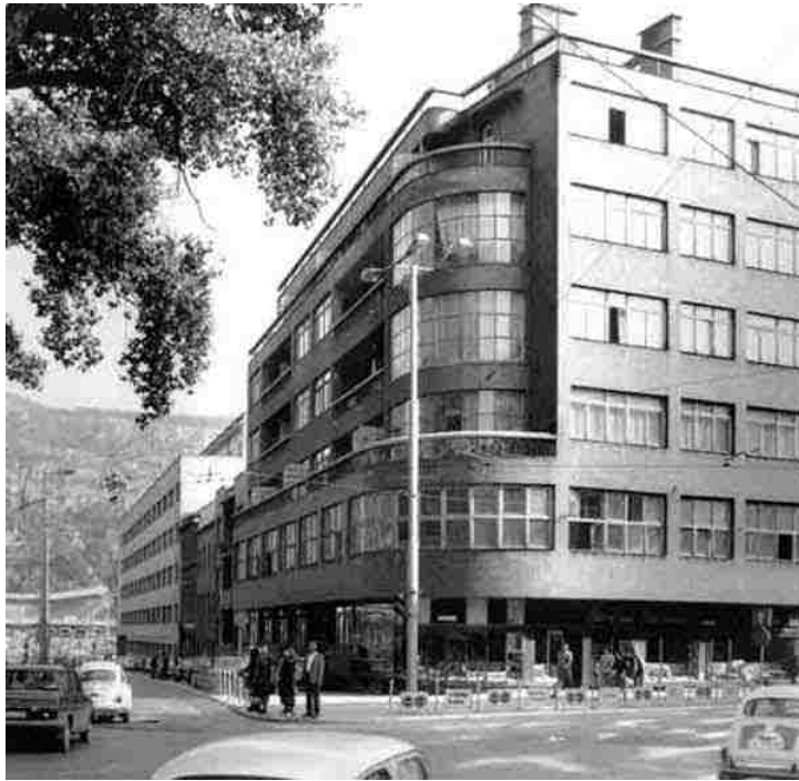
Figure 17: Muhamed and Reuf Kadic, Building of the Pension Fund, Sarajevo, 1940, Courtesy of www.a4a.info
